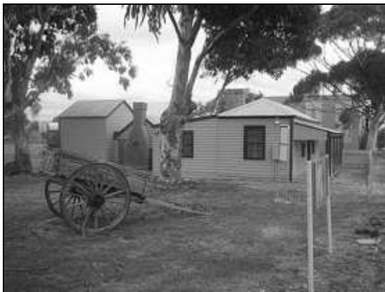
Harrick's Cottage, Harricks Road Keilor 5
