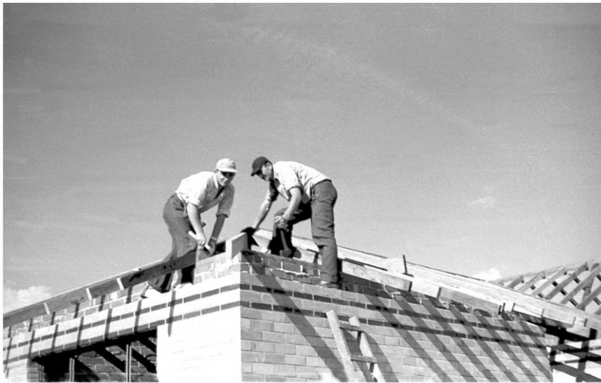
Building the roof, Alfrieda Street St Albans.
