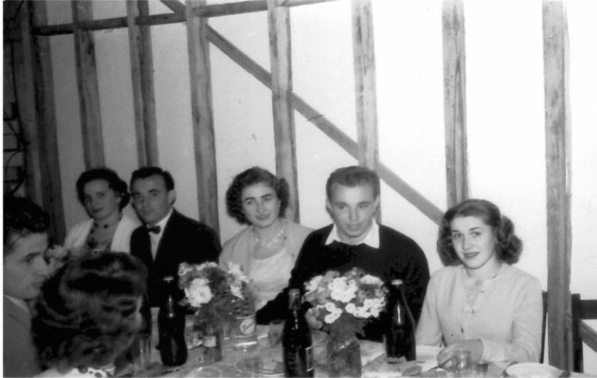
Haumanns and Rossmans celebrating in partly constructed house.
