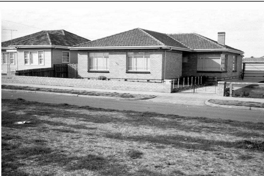
Road and footpath construction, Alfrieda Street, 1957.
