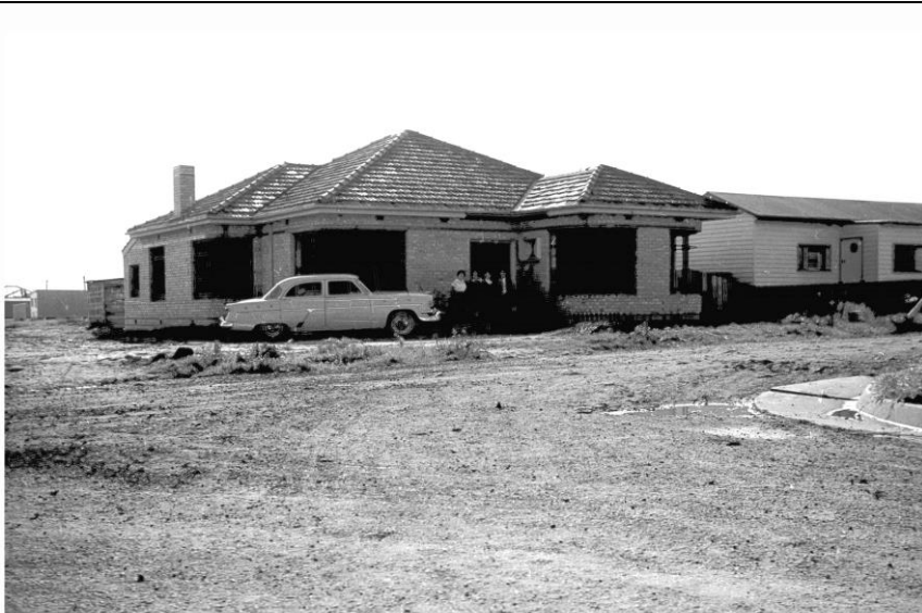
House being built on corner of Walmer Avenue and Station Street.
