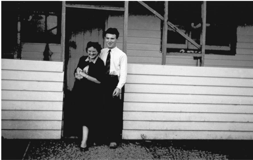
Carl Szabo at house being built in Millawa Avenue St Albans.
