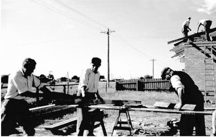
Cutting the rafters for the new house.
