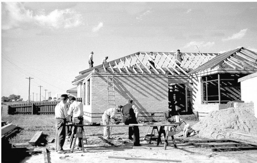
Building the new house, Alfrieda Street St Albans.
