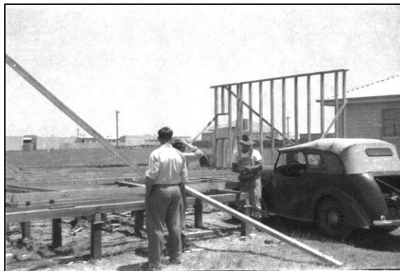
House construction Alfrieda Street © K Haumann
