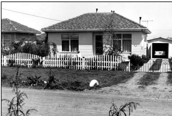
Kivi home in Power Street 1960s © Virve Curtis
