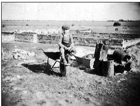
Bernie Kokot on building site 1950s © B Kokot
