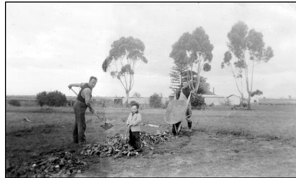
Wilhelm Stein repairing potholes © Mary Smith
